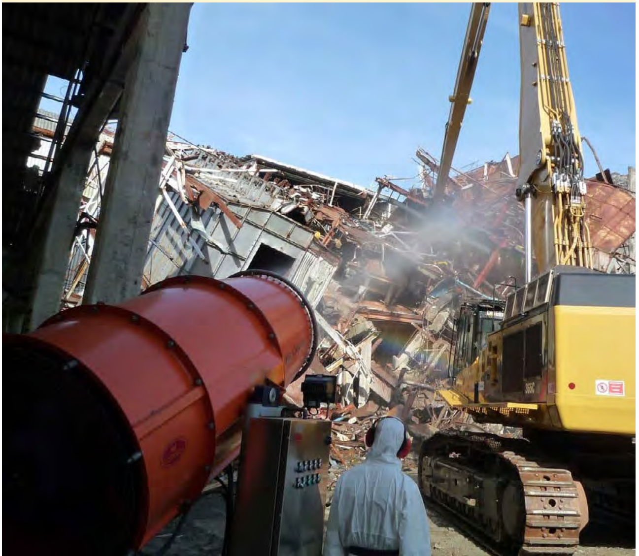
Figure 15-8: Nebulising cannon to dampen dust during demolition of a production plant
