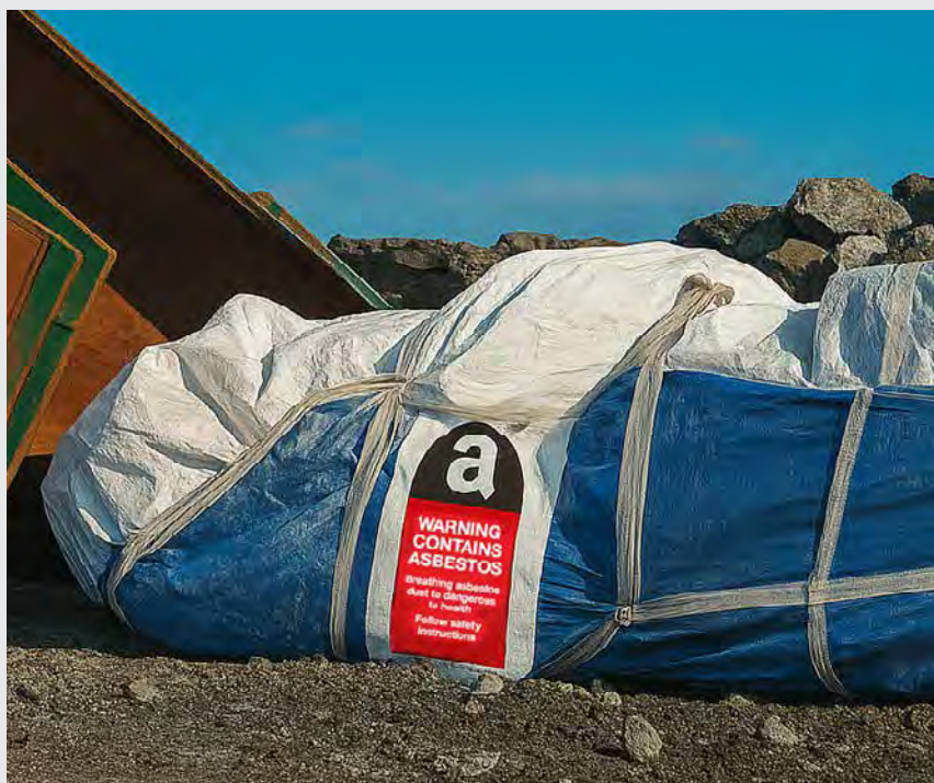
Figure 12-3: WCA disposed in sealed bags
