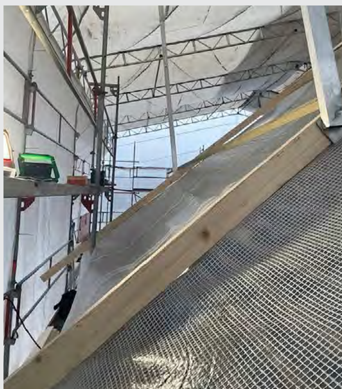
Figure 13-4: Suspension system inside an asbestos tent
