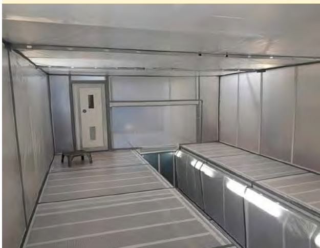
Figure 14-4: Large containment unit with a pit for bogies
