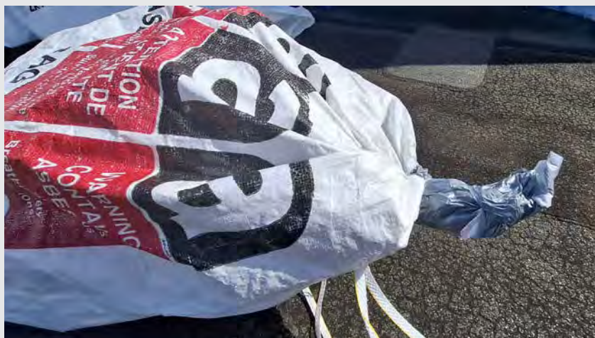
Figure 8-7: Image of a WCA bag tied with a gooseneck closure
