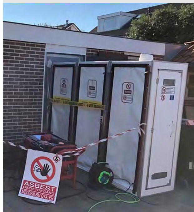
Figure 8-5: Example of a decontamination unit set-up
